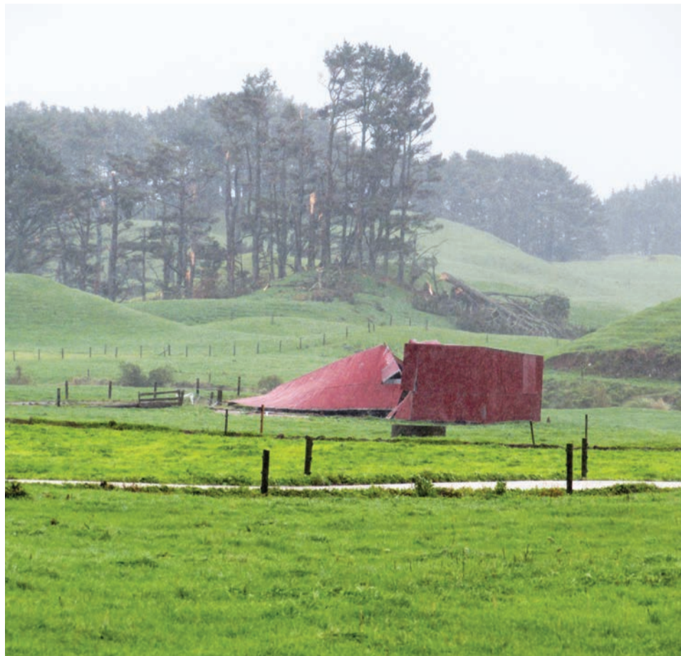
The aftermath of the storm.
