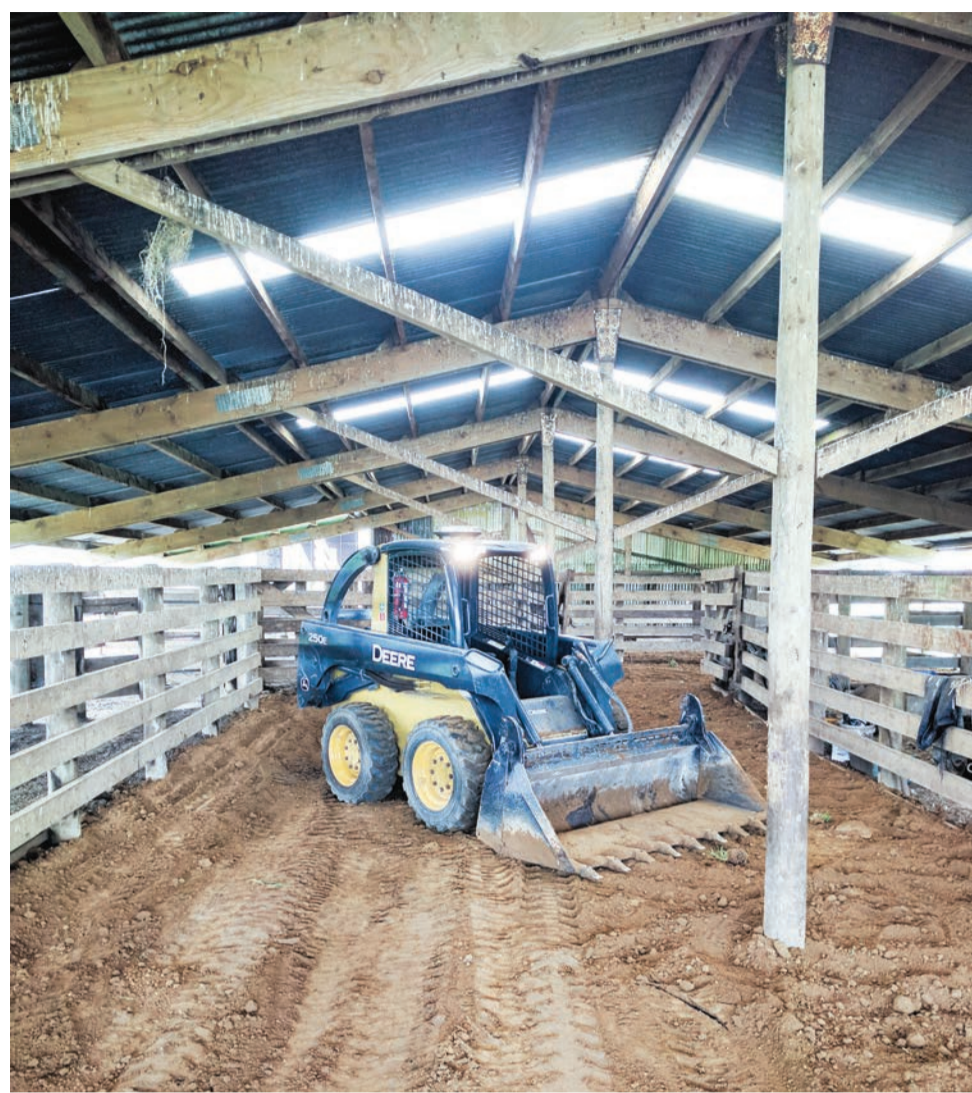
Good modern gear means Excavat can get to places where others cant.
