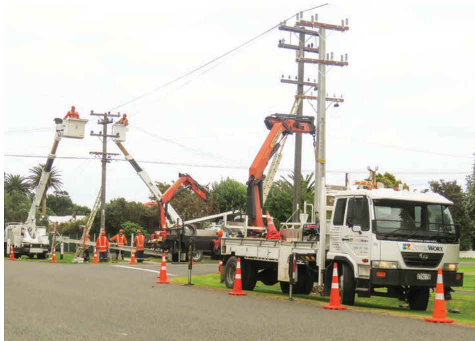
Powerworx replacing power poles in Layard Street, Opunake.
