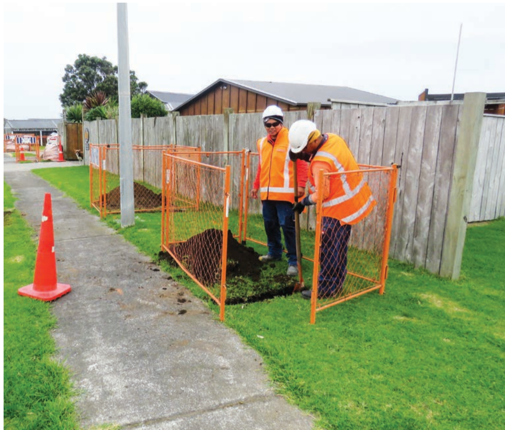
Laying fibre optic cable, beginning in Hickey Place at the northern end of the town.
