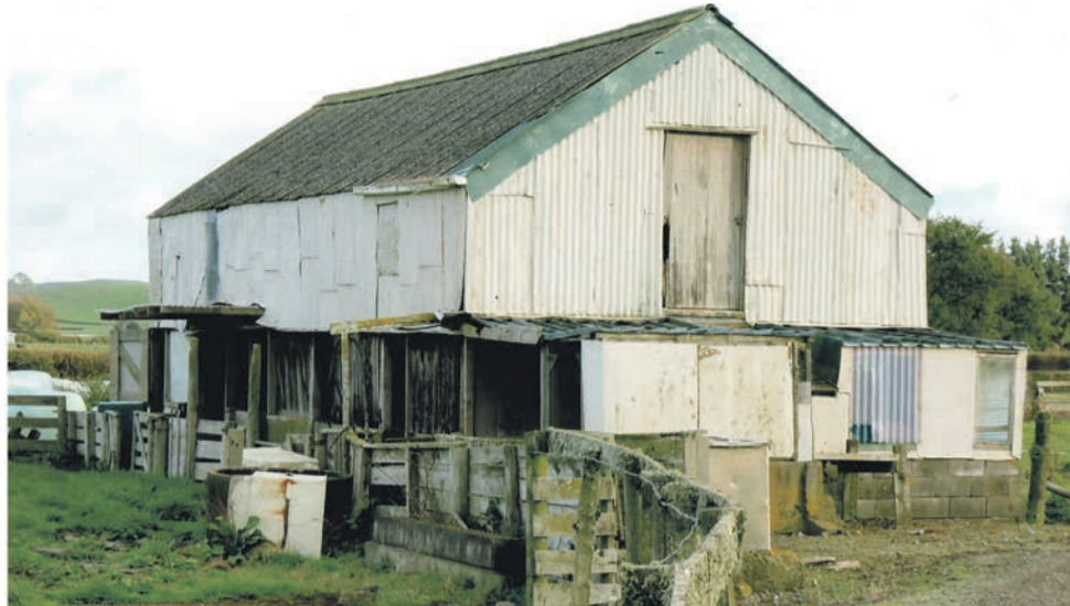
The 1943 piggery at Routh Carr, Eltham showing the corrugated iron covering the old tarred wallboards.
